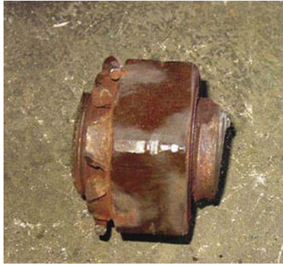
Figure 2. Location of fatigue fracture in a change of section on the pump shaft.
