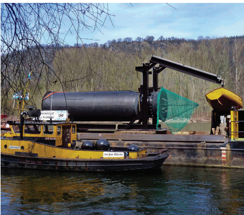
Installation of a river turbine made by KSB in an arm of the river Rhine at St.Goar.
