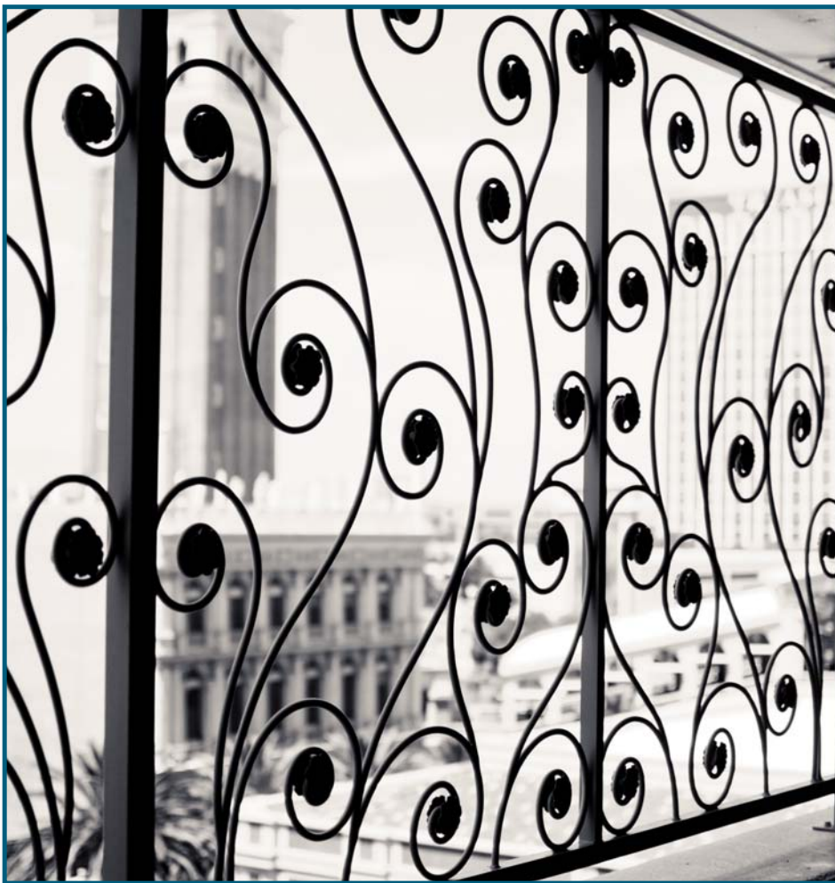
The installation AR Iron completed for the garage structure at the Venetian Resort Hotel & Casino entailed 8,000 hand-forged solid bar scrolls complemented by 16,000 deco rosettes attached to the finials. The entire job, which spanned eight parking levels, took 90 days.
