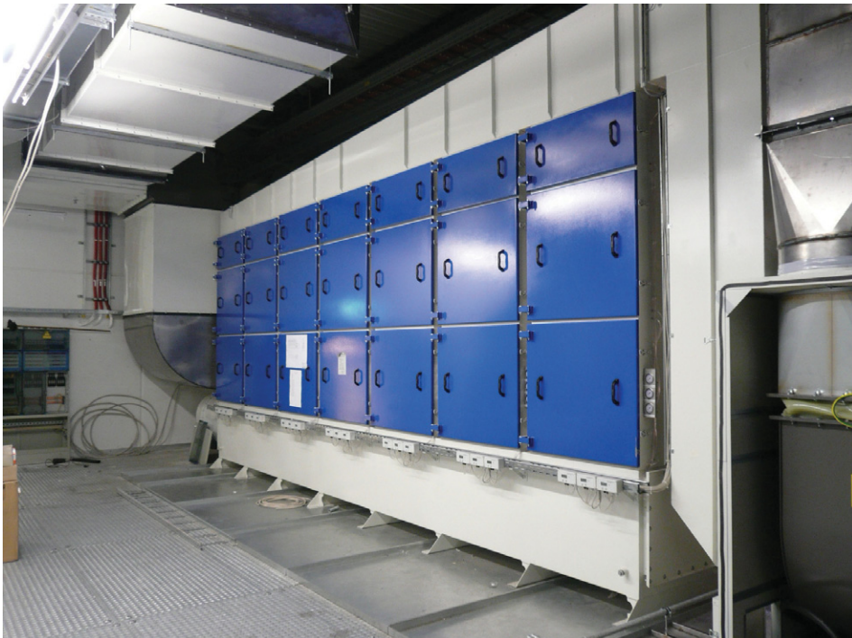
Figure 2: Oil mist elimination system for a German automotive manufacturer. (Courtesy of Vokes Air Group.)
