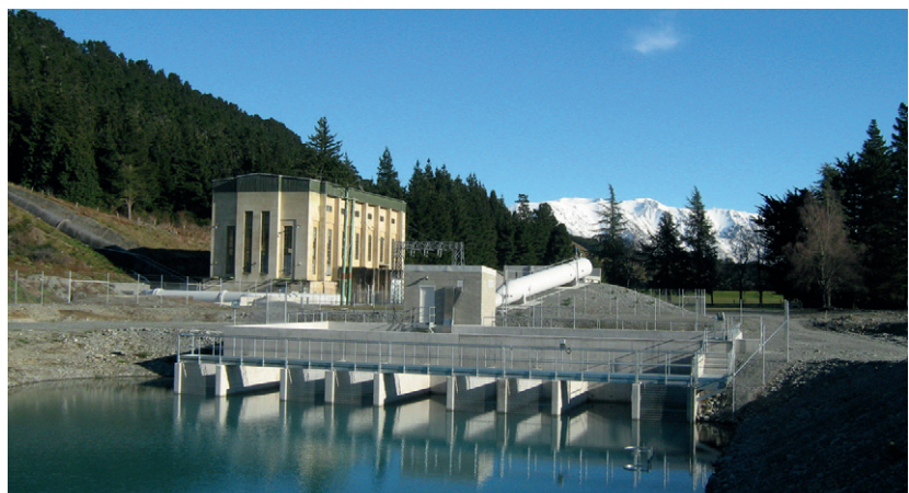
TrustPower Highbank power station and new pumping station located on the Rakaia River in New Zealand's South Island.
