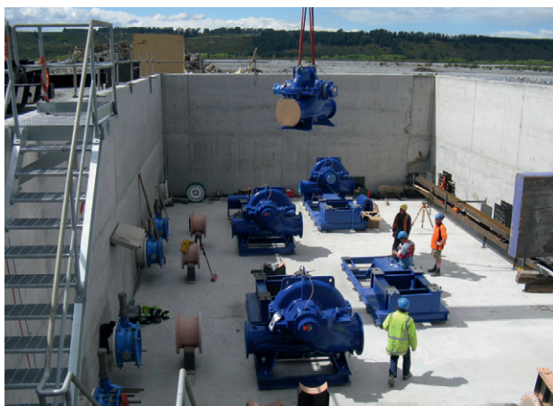
Delivering the five KSB RDLO 500-800Aw 1500Kw pumps.
