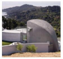
Kreysler's award-winning California Bay House is a monocoque structure consisting of nine custom-moulded, fire-retardant FRP sandwich panels.
