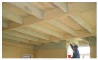
InnoVida FCP panels are joined using InnoVida Bond, which forms strong chemical welds, eliminating the need for fasteners such as screws and nails.
