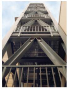
This 63 ft (19.2 m) freestanding stair tower was constructed using Strongwell's Extren® structural components.
