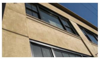
Simulated stone exterior trim features a polymer concrete face coat backed with FRP sheets on this Kreysler project.
