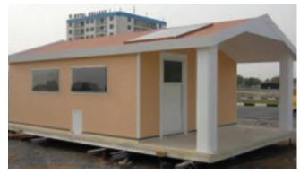
A standard house can be constructed using prefabricated InnoVida load-bearing, insulated FCP panels in 1-3 days.
