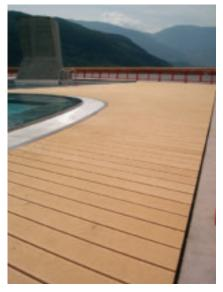
Tech-Wood WPC decking, reinforced with oriented long fibres, is said to provide high bending stiffness and strength.
