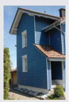
This house was built using Tech-Wood's WPC siding, developed in cooperation with extruder manufacturer Cincinnati Extrusion.
