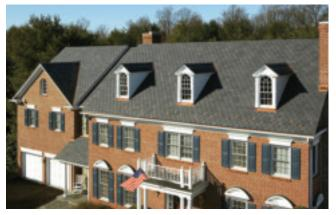
Composite slate roofing shingles from CertainTeed are lighter and more durable than natural slate, with a much less expensive installed cost.
