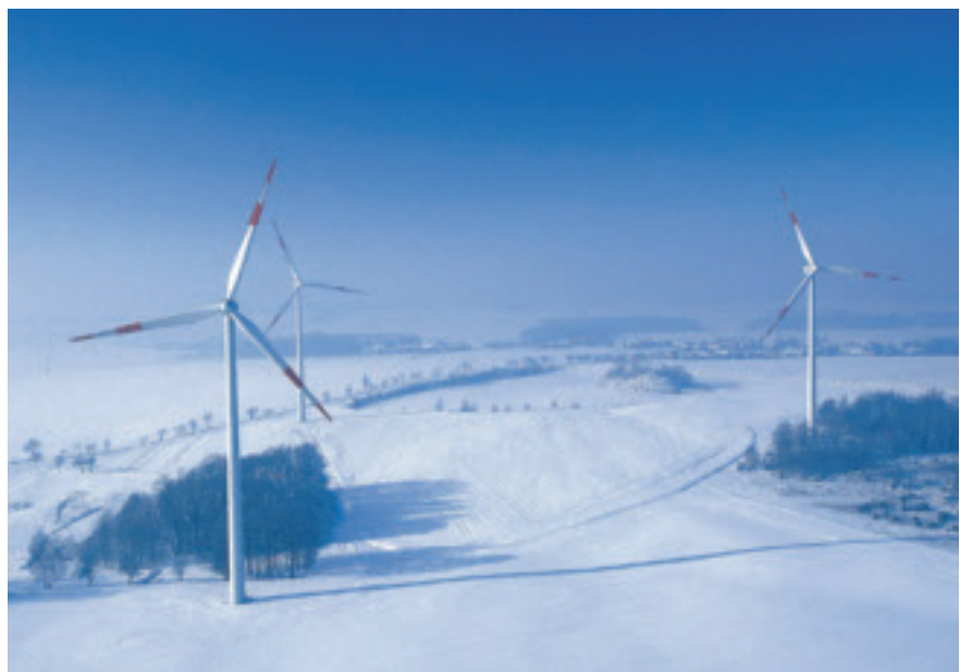
FRP components must be durable enough to stand up to harsh weather such as seen in this picture of Vestas wind turbines during winter in Germany. (Picture courtesy of Vestas Wind Systems.)
