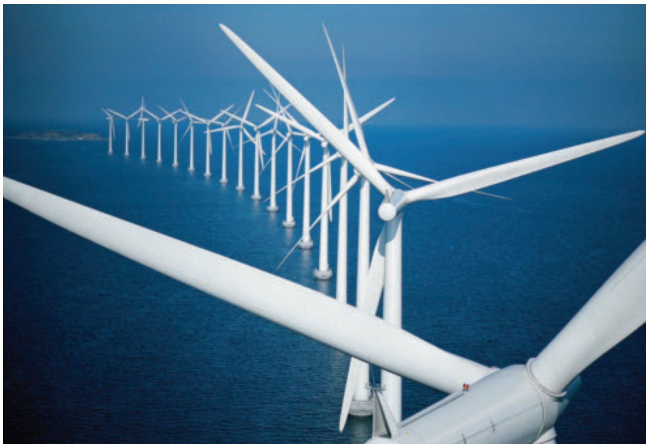
Offshore wind farm with 22 Bonus Siemens wind turbines fitted with LM 26.8 m blades. (Picture courtesy of LM Wind Power.)
